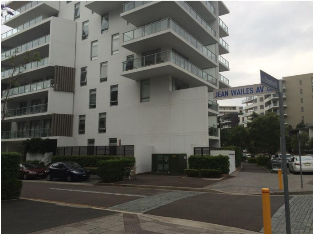
Figure 2 – Example of the poor design outcome achieved when a substation is placed in front of a building, requiring a 6m blast zone
