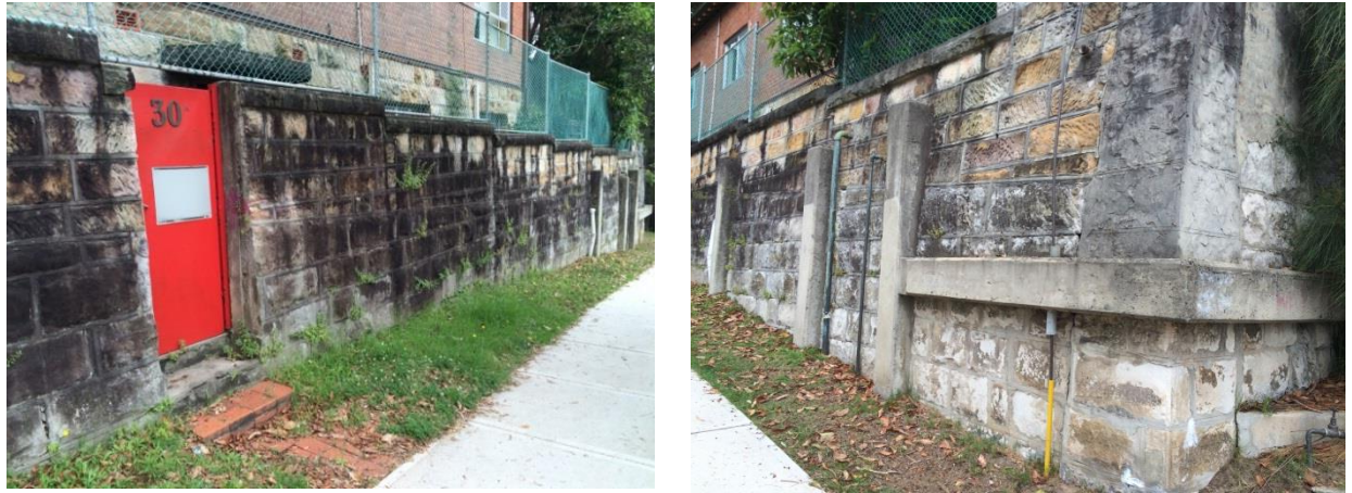
Figure 8 – View of the sandstone wall on Wellington Street, showing the existing opening and the wall's poor state of repair
